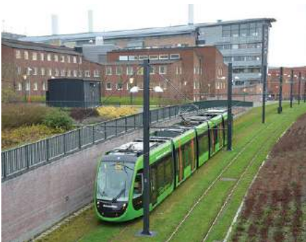
▲ ABOVE: The underpass at Tornavägen was built for the busway in 2002, featuring a nice brick wall design.
