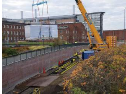
▲ ABOVE: The tramway's second substation is lifted into place on 4 November 2018.
